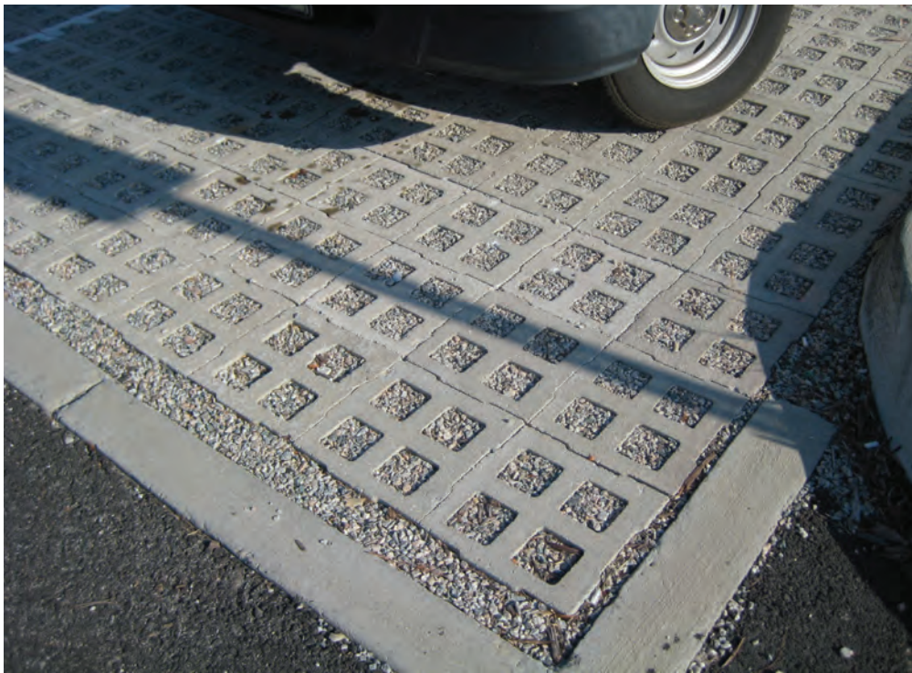
Figure 3.3. Permeable paver parking installation, light commercial scale. (Source: New York State Stormwater Green Infrastructure)
