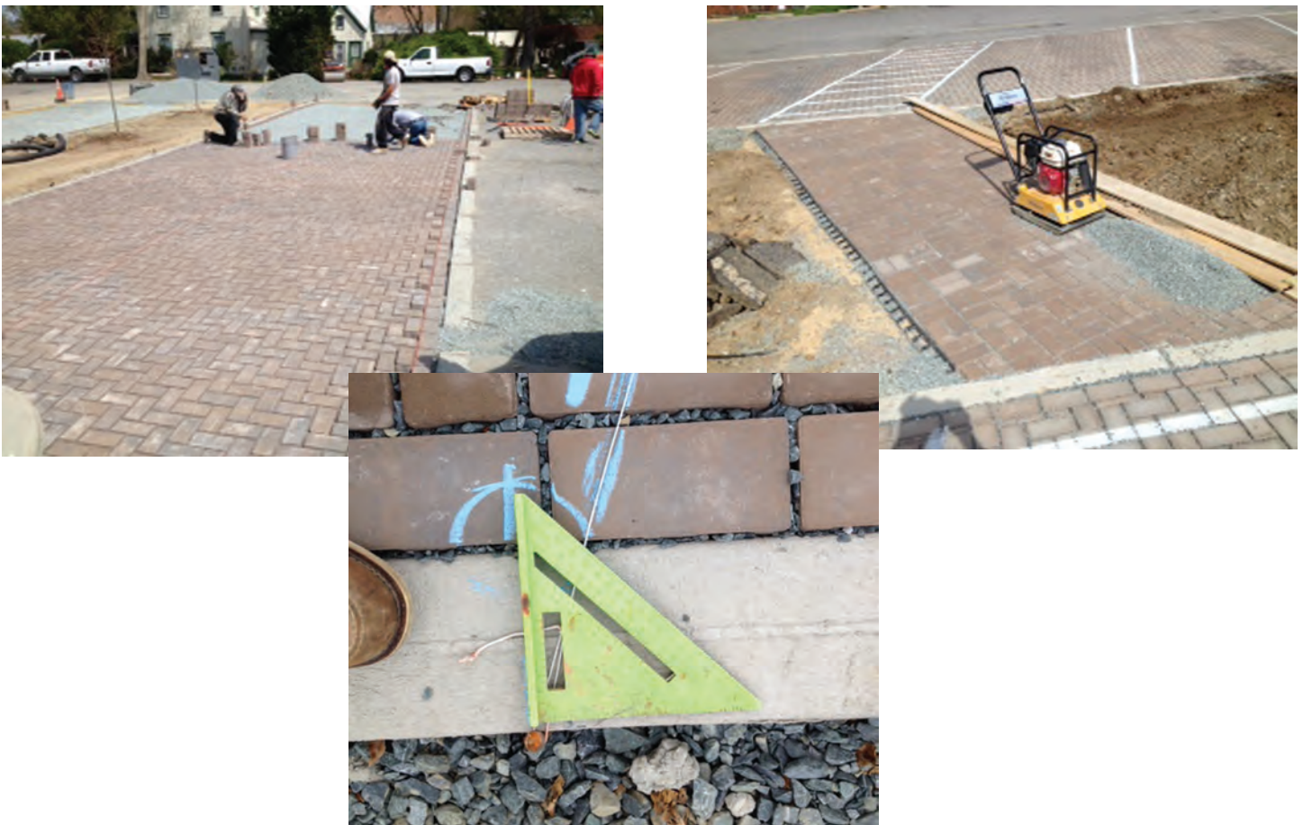
Figure 3.10. Installation of pavers (top left), compaction (top right), and filling spaces with pea gravel (bottom).
