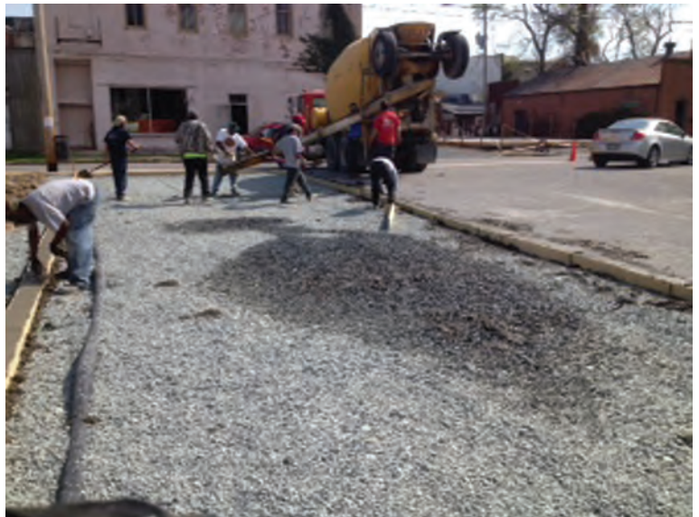
Figure 3.9. Installation of gravel reservoir layer
