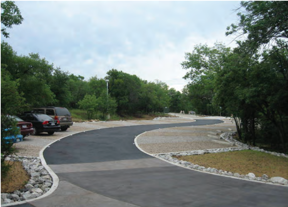
Figure 3.7. Gravel diaphragm and grass filter strips to catch sediment before runoff reaches permeable pavement
